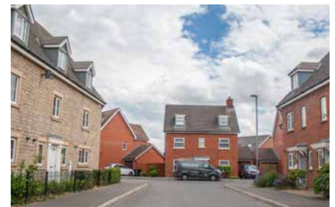
Residential development in Calverton
