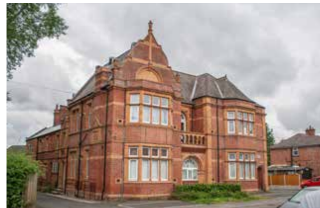
Bestwood with its grid layout, terraces and landmark buildings that supported the colliery industry
